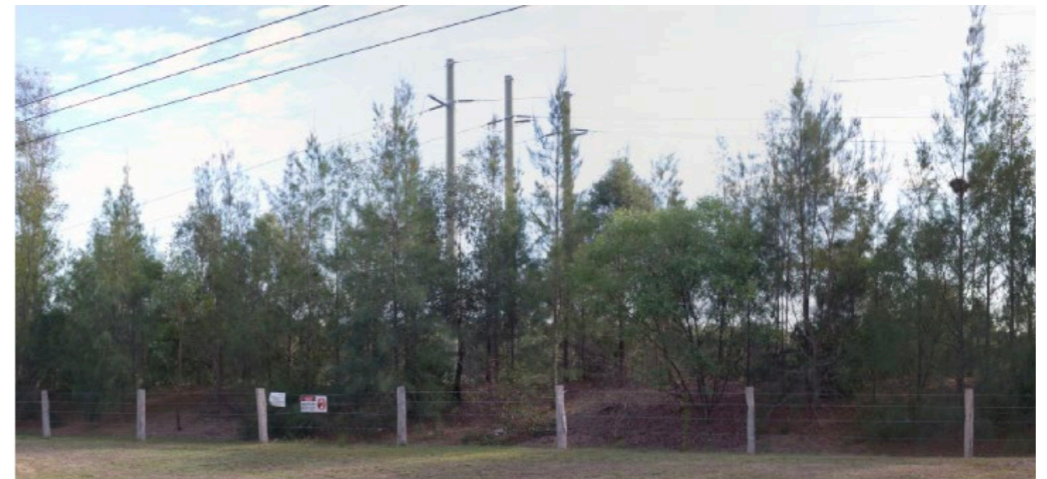
Image 31. Example of screen planting to mitigate a substation
