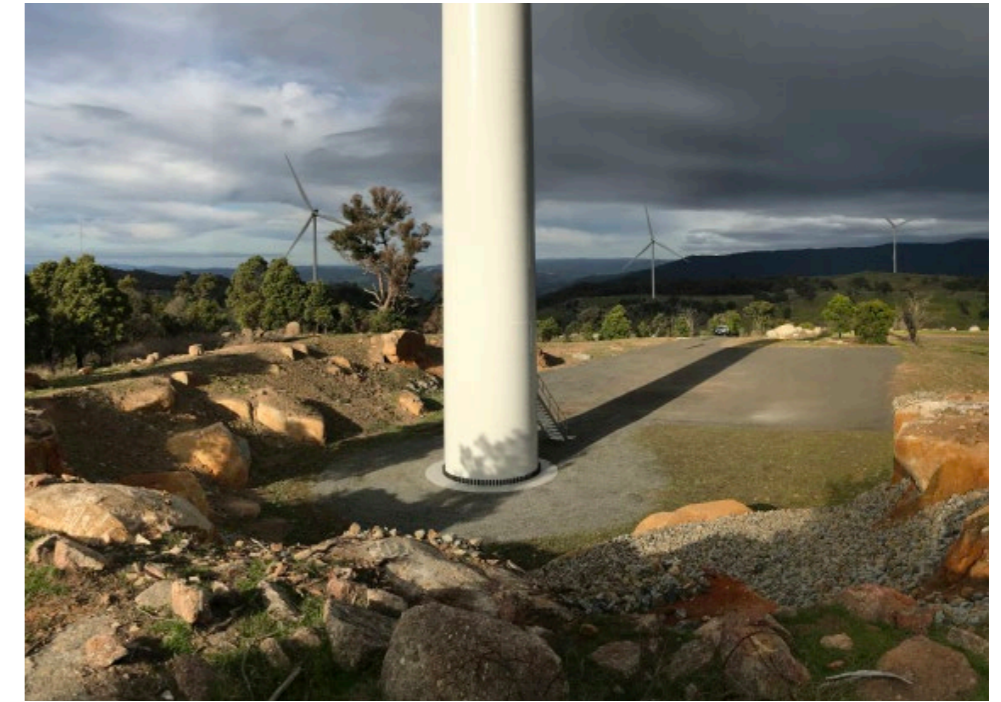
Image 3 Crane Hardstand Area (Source: NGH)
